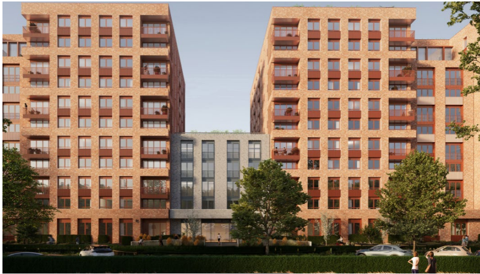
Figure 5 – Five storey high link blocks
