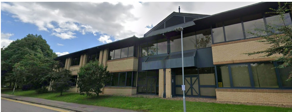
Figure 17 – Existing site frontage with Napier Road
