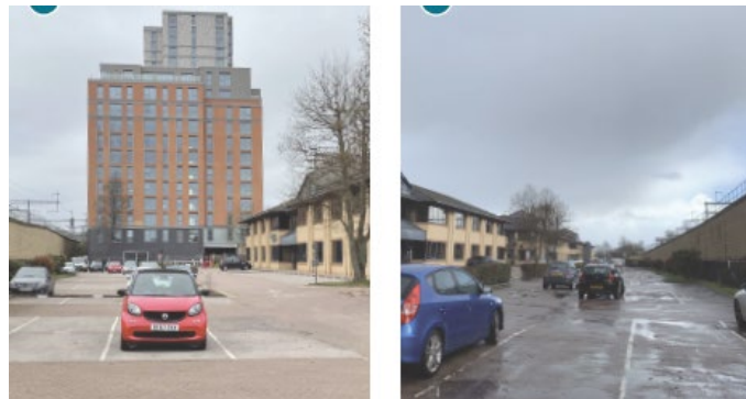
Figure 18 – Existing view looking west and east from the rear car park showing the Network Rail retaining wall
