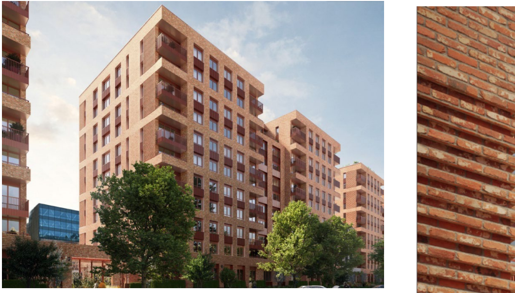
Figure 42 – Visual showing side elevations of the blocks and close up of the feature brick panel bands of projecting brick courses
