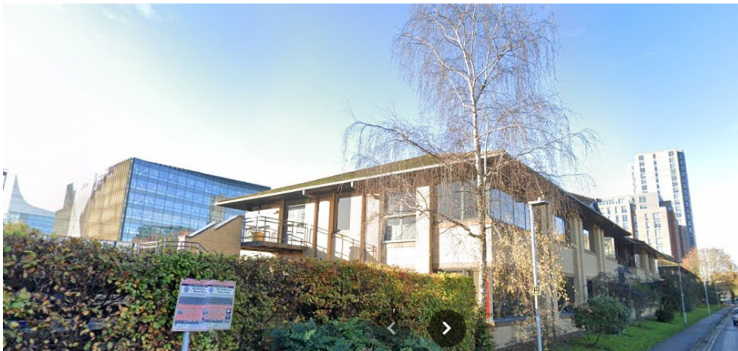
Figure 29 – Existing view looking west along Napier Road
